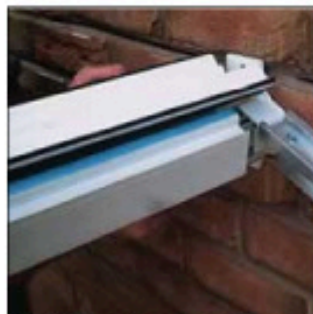
3. Ridge beam slots onto wall hanger
