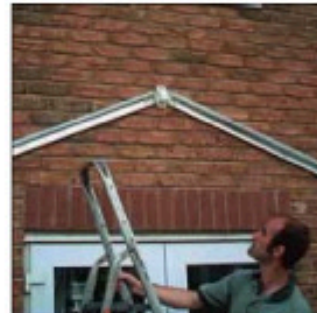
2. Getting the 'A' frame into place
