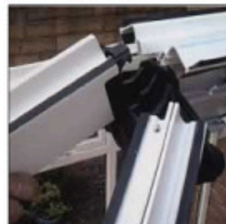
4. Glazing bars just click into place
